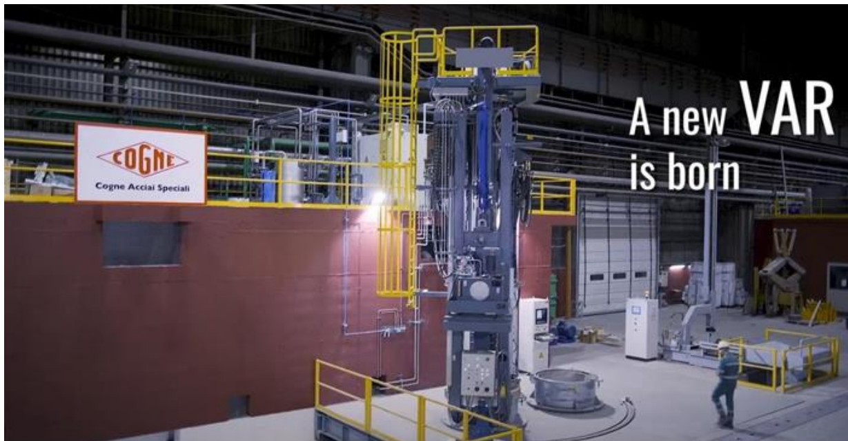
Figure 2. New VAR plant
